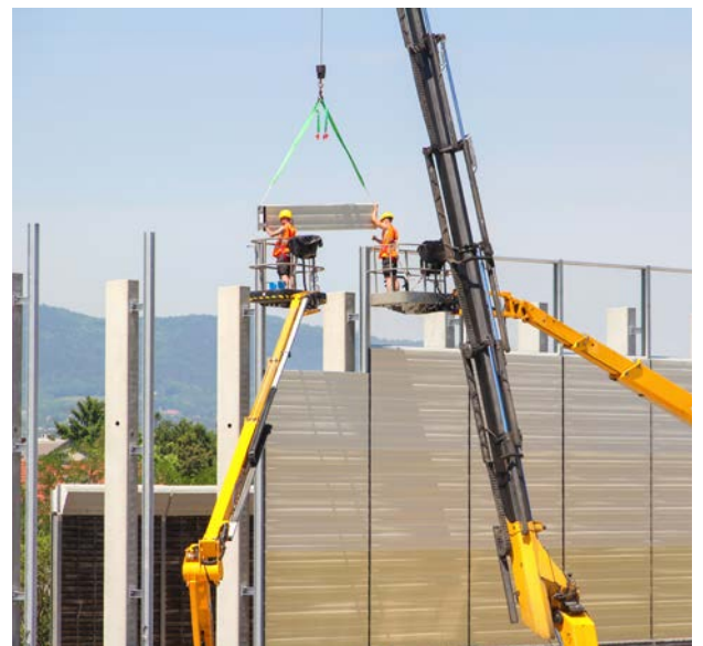
The fitters need to overcome dizzying heights.
