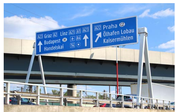
Static direction signs on a Flexgantry bridge.
