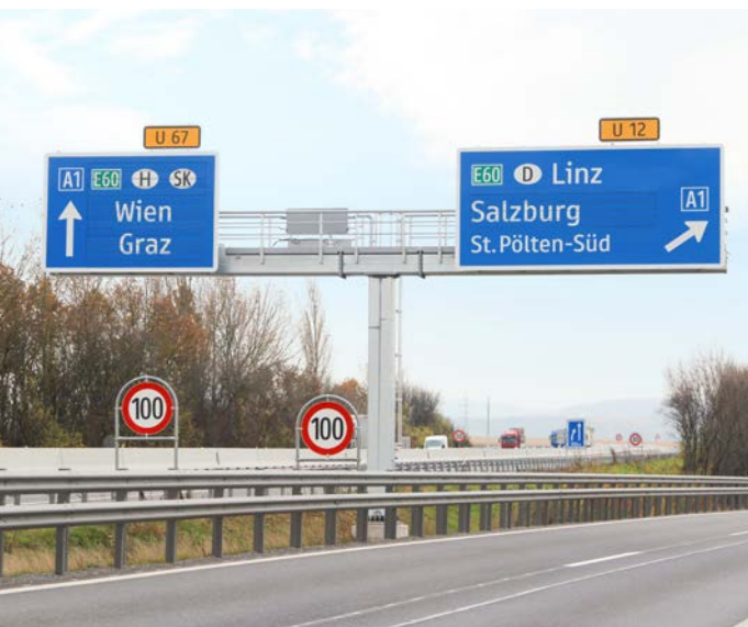
Prism-type variable traffic signs mounted on a T-shaped suspension pole.
