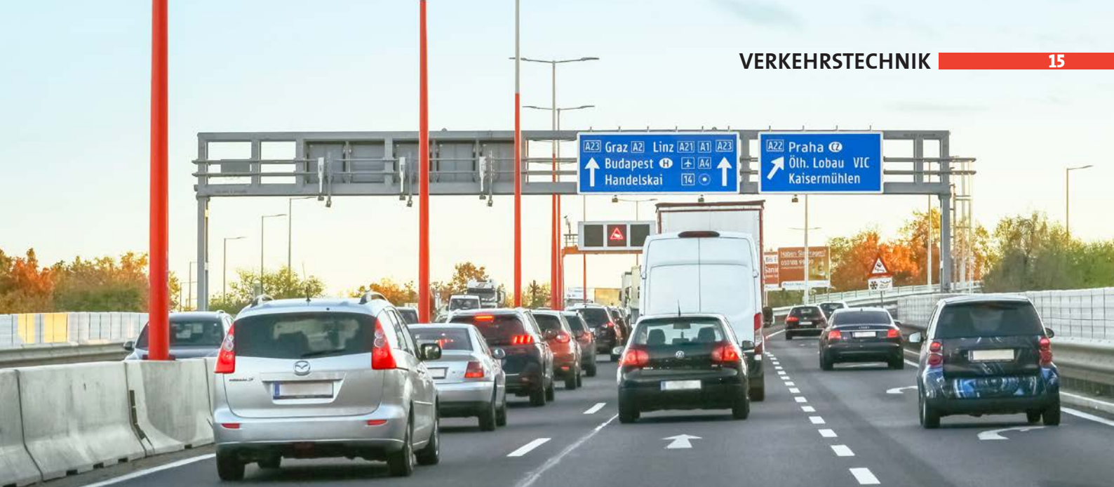
Truss bridge for traffic signs.
