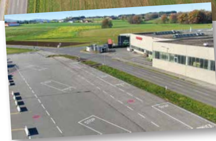
The new lorry loading and unloading zone.
