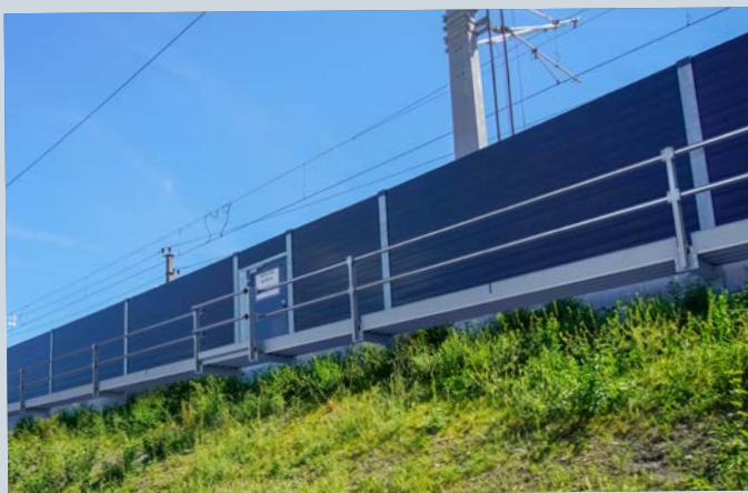
The FONOCON inspection catwalk facilitates access to difficult-to-reach spots along a railway track.
