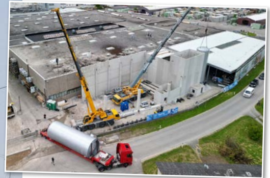
The buffers (capacity: 105,000 litres each) were put in place in the summer of 2024.
