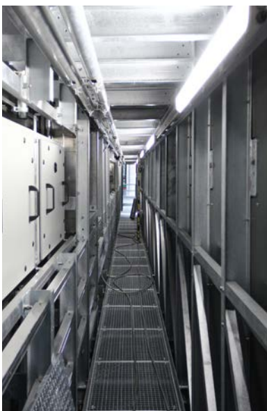
A view inside the gantry.
